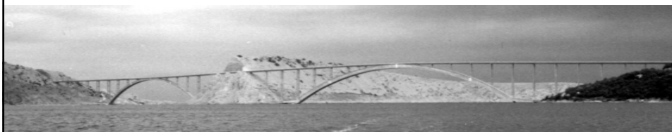
Krčki most – prevodi naftovod
