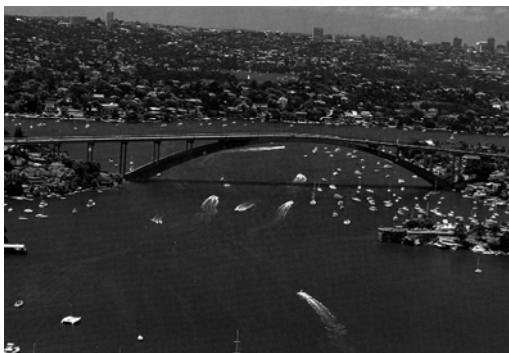
plovidba ispod mosta Gladesville u Sydneyu
